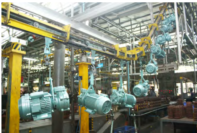
Conveyorised Pump Assembly
